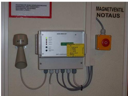
O<sub>2</sub>-Control panel in the basement opposite to the filling station with alarm horn (left) and red emergency shut-off button (at right) for liquid nitrogen line.
