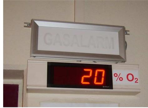
Display besides the stair case on the ground floor showing the oxygen content in front of the liquid-nitrogen filling station in the basement.
