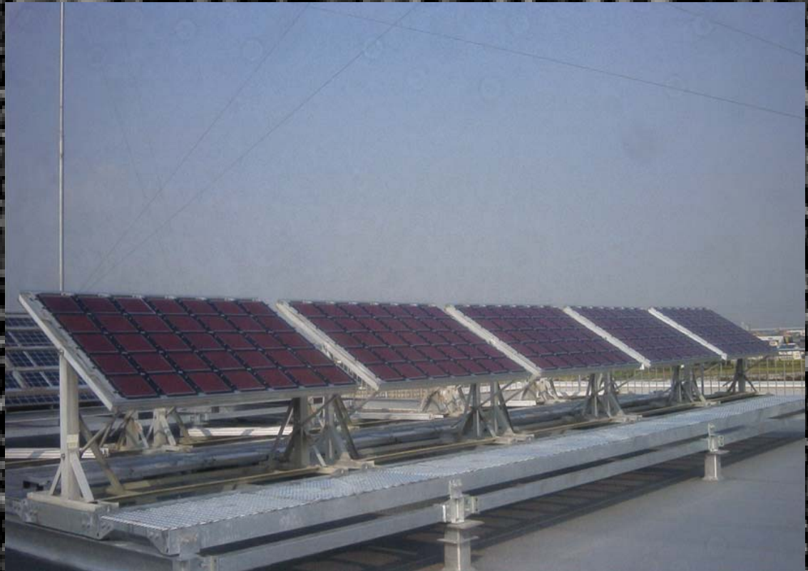
Kariya City at lat. 35^{\circ}10'N , Asimuthal angle: 0^{\circ} Facing due south, Tilted at 30^{\circ}
