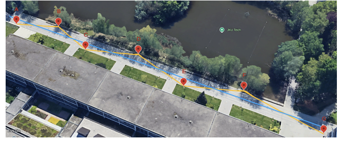
Fig. 2: Bird view of the experiment scenario(180x8m)(taken from Google Earth). The red markers indicate the key points, the yellow line represents the intended trajectory for the participants and the blue line exhibits the intended trajectory for the vehicle.
